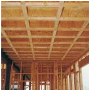
Origin™ I-floor supplemented with noggings to achieve fire rating as per Gib® Fire Rated Systems.
